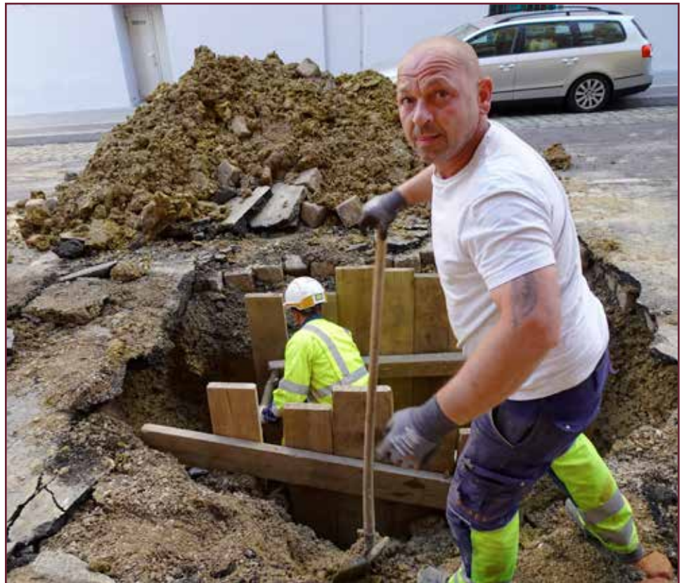
Workers for Wiener Wasser (Vienna Waterworks) digging to find the break.
